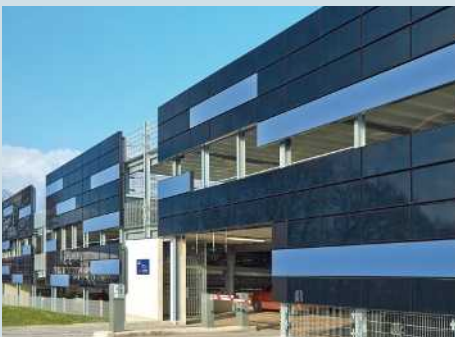
Building-integrated photovoltaics (BIPV)
