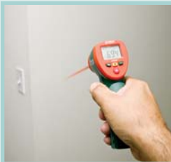
Check building for insufficient insulation
