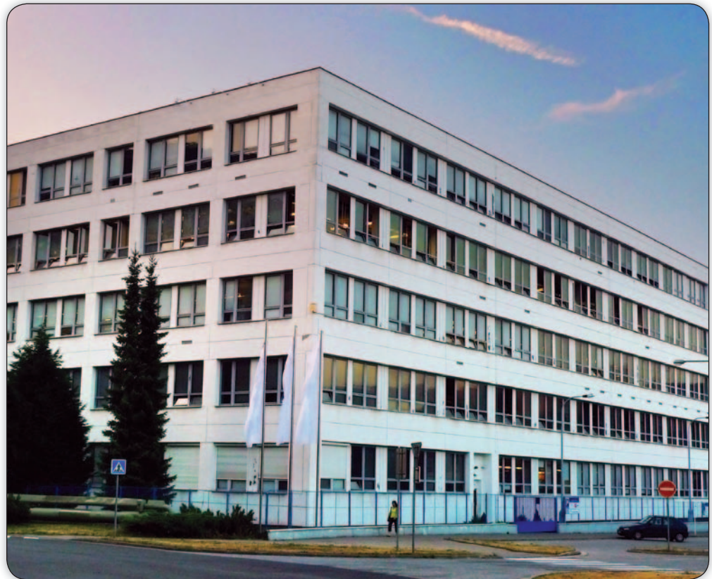
TE Manufacturing Facility in Trutnov, Czech Republic
