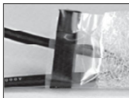
**3.7 Seal Mold.** Starting at bottom of mold, seal and compress sealing mastic around and between each cable to form a resin tight seal.
