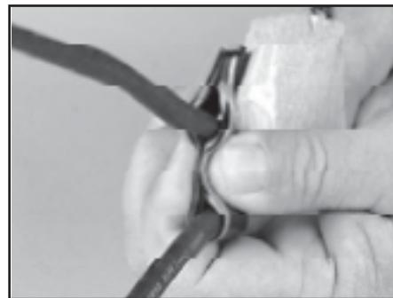
**3.8 Level Splice.** Ensure that top of mold is level. If support is needed, support the cable outside of the splice area.
