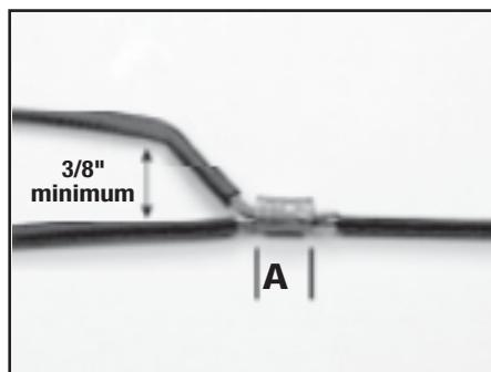
**3.3 Train Cables.** Place cables in a horizontal position. Spread legs of cable so there will be 3/8" space between cables to allow for sealing around each cable with mastic sealing strips.
