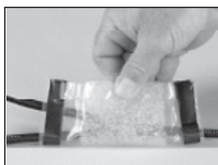
**3.6 Seal Film.** Seal film together between spacer pad and mastic.
