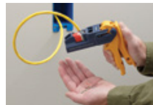
6. Wires will be seated and cut for a solid termination.
