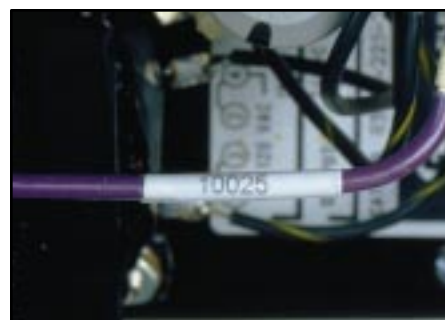
Immediately apply self-laminating labels
