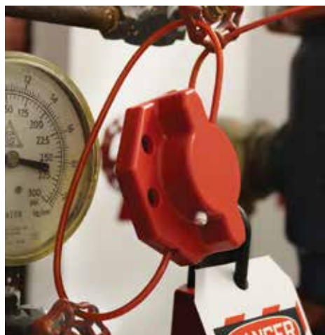
Turn the hasp halves to cinch cable.
