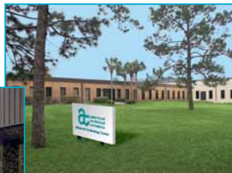
▲ ATC's Jacksonville Facility occupies approximately 100,000 sq. ft.
